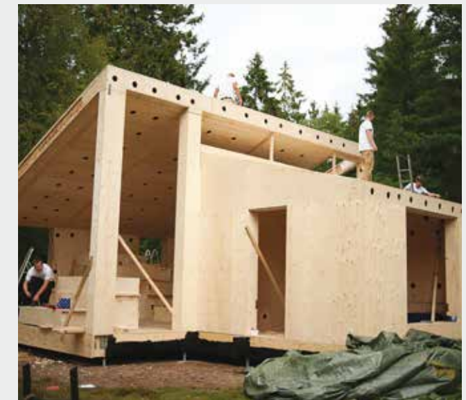
Building in a Snap. Danish company Eentileen and Facit Homes collaborated on Villa Asserbo, a digitally-fabricated cottage. Parts were "printed" from sustainably-harvested plywood using a CNC machine, then snapped together.
