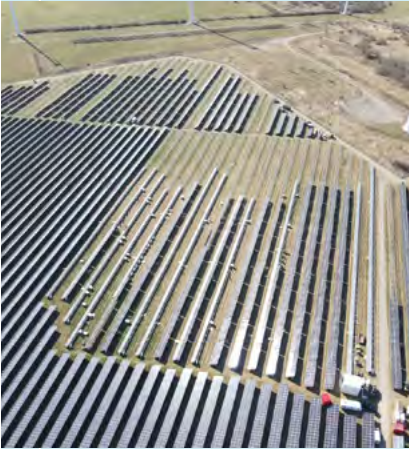
During the conversion
