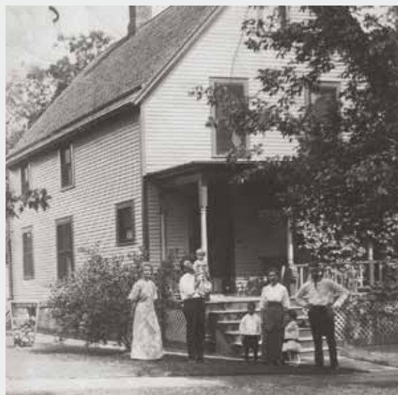
Full Circle. The Grocoffs’ historic home did not originally depend on centralized water and sewer infrastructure.
